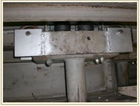
Many hangar door companies provide doorstop bumpers within the top track assemblies. The problem with situating bumpers in the top rails is that the loads required to stop a big door section is tremendously high. The building supplier normally does NOT account for this load. Spec-Dor provides doorstop bumpers that are at the end of the bottom rails.
