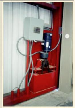
signed correctly, the sheer inertia of the door weight can destroy the gearbox.
